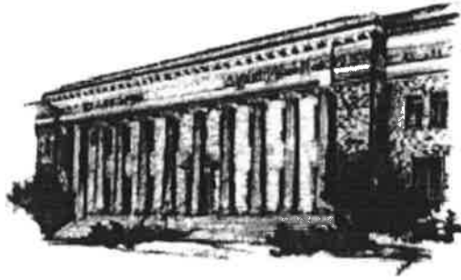
Tehama County Courthouse
